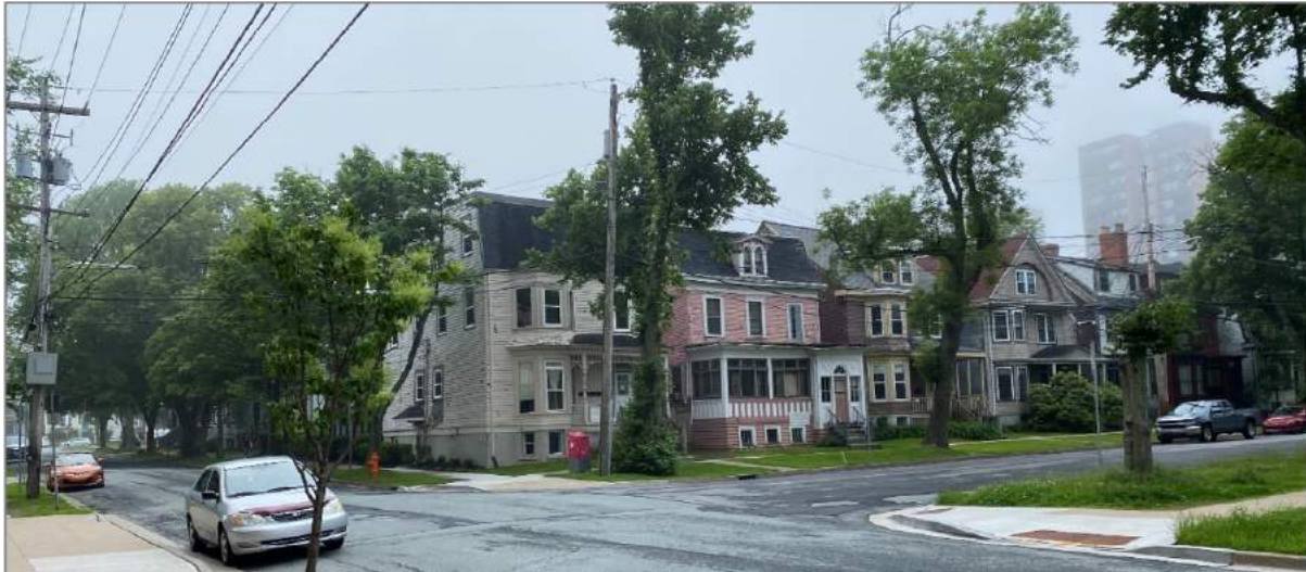
Some of the houses in the Carlton Block that would be demolished to make way for new highrises if the HRM Council approves the development project. (Photo: Heritage Advisory Committee) 21
